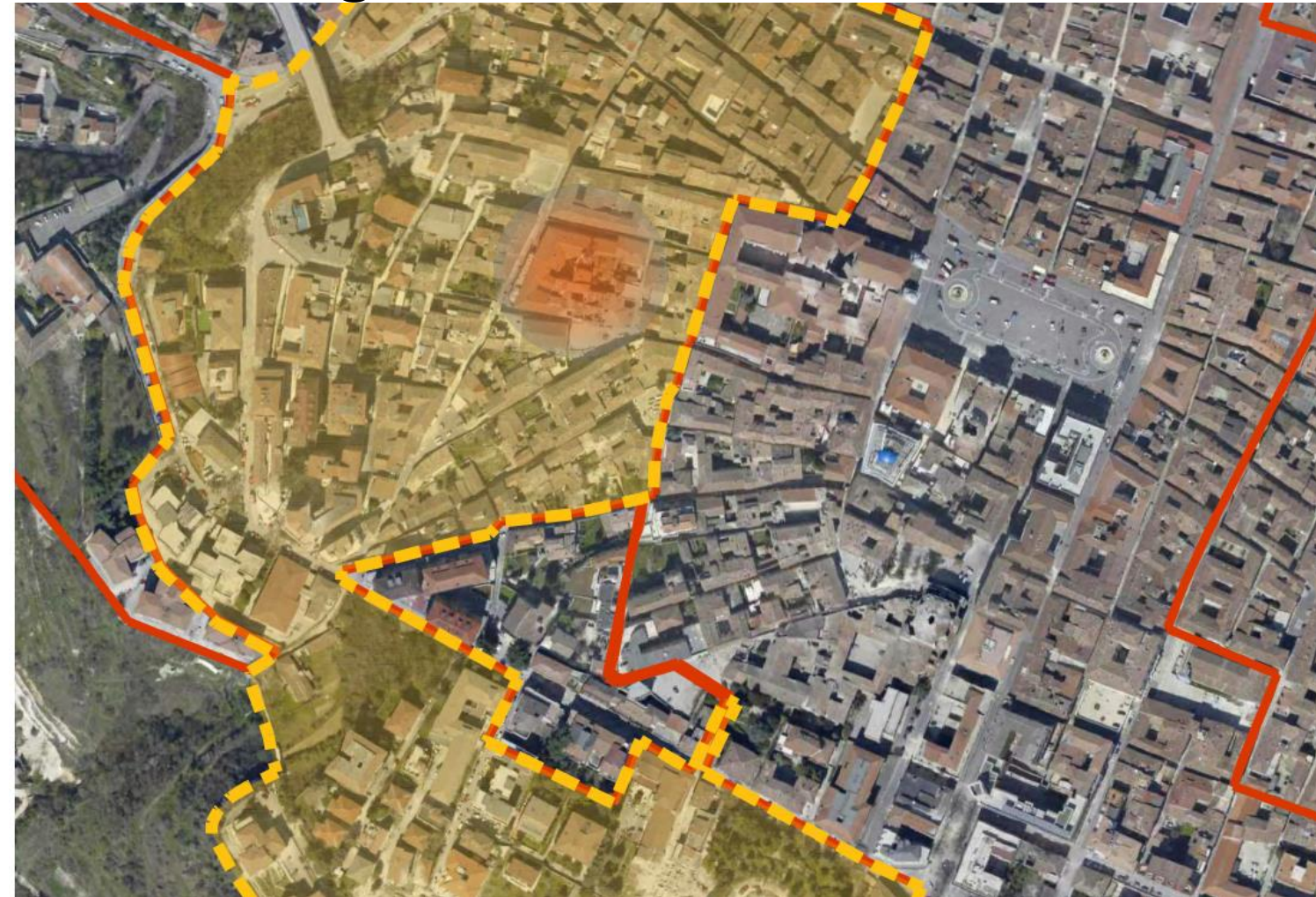
In ORANGE , the aggregate for which the repair, structural seismic improvement and restoration project was drawn up is highlighted - AERIAL PHOTO
